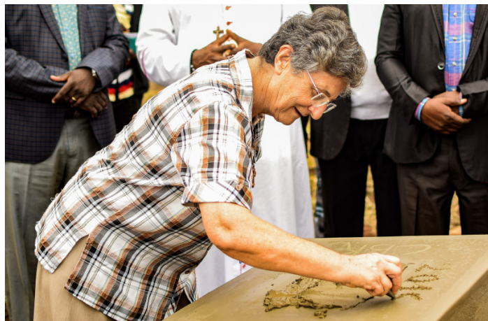
Sister Laura is the hospital administrator at St. Theresa Hospital. She marks the date of the ground breaking on the ceremonial first brick.
